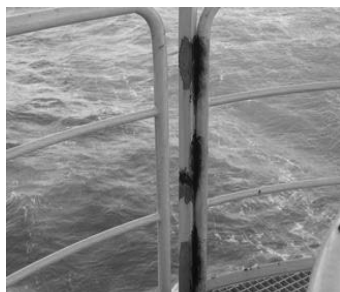
Coating deterioration
