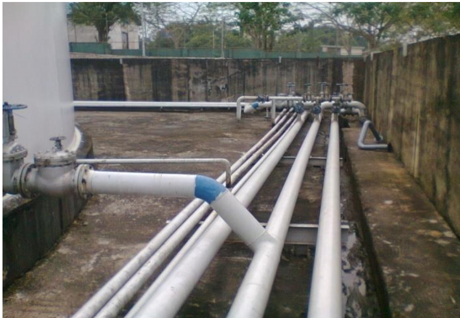
Figure 9: Painted Pipelines in the Tank Farm, with colour codes for specific products
