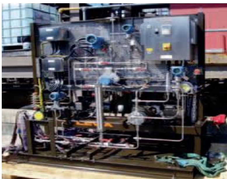
Figure 15: The 'highly reliable chemical injection system' deployed at the refinery, providing real-time data to a unique piece of software that helps field personnel manage corrosion more effectively. 9
