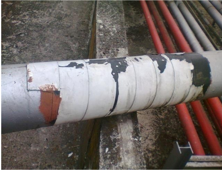
Figure 10: Epoxy Wrapper on Pipe Section across a Bundwall
